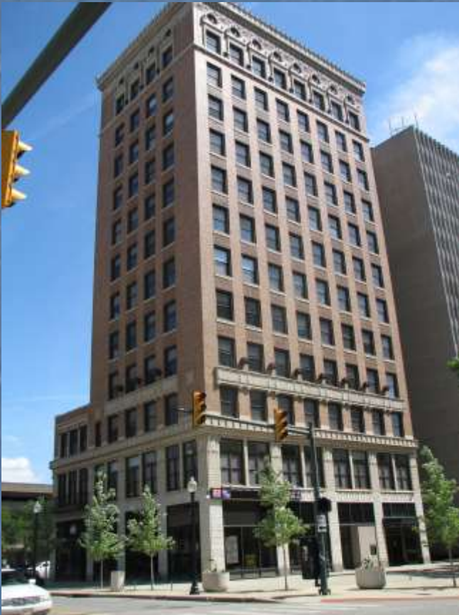
Historic Office Building Converted to Apartments
